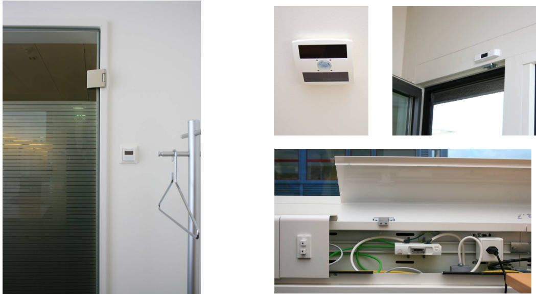
Figure 2-2: Additional equipment installed in offices: wireless room temperature sensor (left, next to the office door), wireless presence and illuminance sensor (top middle, at ceiling), wireless window contacts (top right, above the window), electrical energy meter for measuring consumption of electrical lighting (bottom right, within the media channel).
