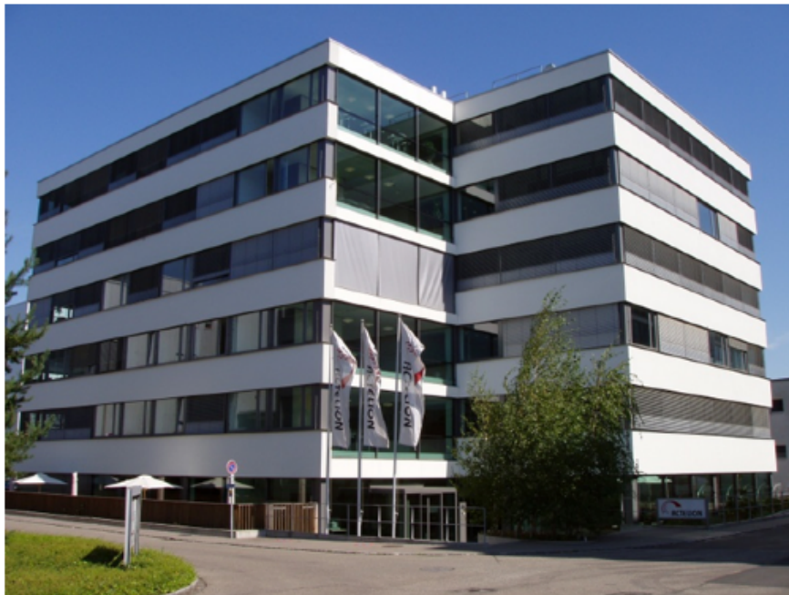
Figure 1-1: View of the target building from the south
