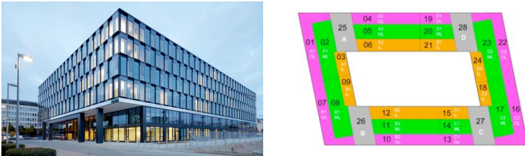
Fig. 2: View of the Icade Premier House 1 (Munich); used zoning of the third floor.
